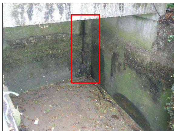
Figure 3-13 Flapped outfall from balancing storage in north-west corner of site
