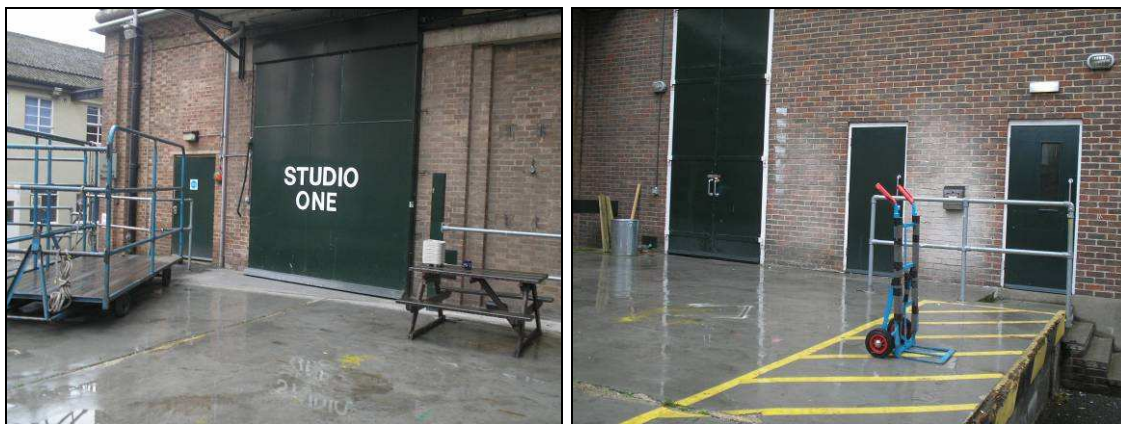
Figure 4-14 Selection of doorways and access points to buildings on the site
