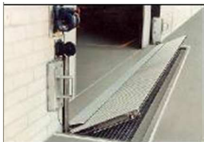
Figure 4-3 Example of suitable “Flip-Up” Flood Barrier
