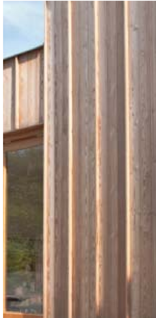
Vertical timber boarding for top floor
