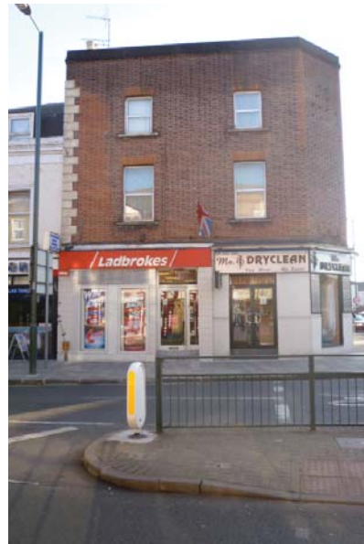
Views of existing buildings
