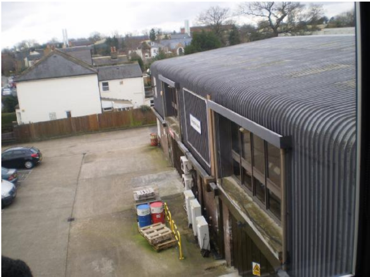
View of gable of No. 8 Queens Road taken from second floor window at rear of Existing Office property; looking South; showing the setback of the office building return behind the 2 storey return of No. 8 Queens Road.
