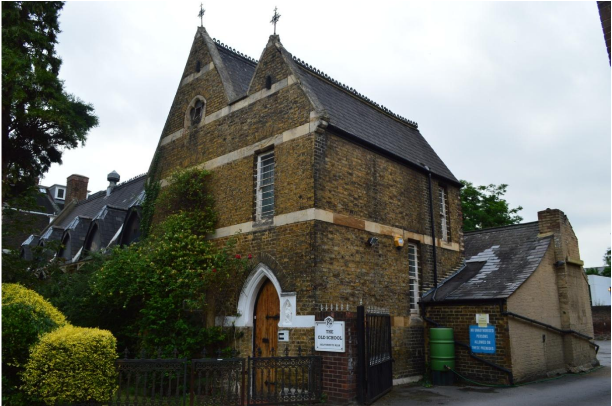
View from the south east, showing the master's house with its single storey ancillary wing to the right, and the dormer windows of the original school hall on the left.
