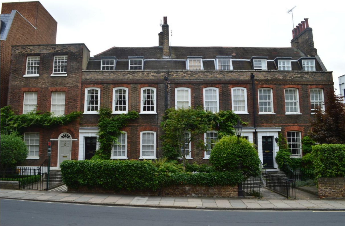
The listed early Georgian houses at 3, 4, 5 and 6 Parkshot. The modern office block at Nos. 1 & 2 can just be seen to the left, with the edge of the Magistrates Court on the right.
