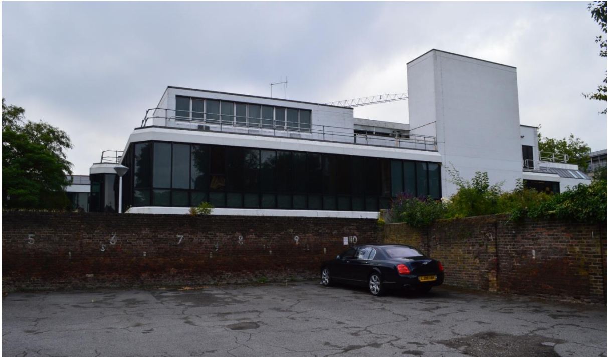
View north from the Old School site, showing the Brutalist white-painted concrete Magistrates Court.
