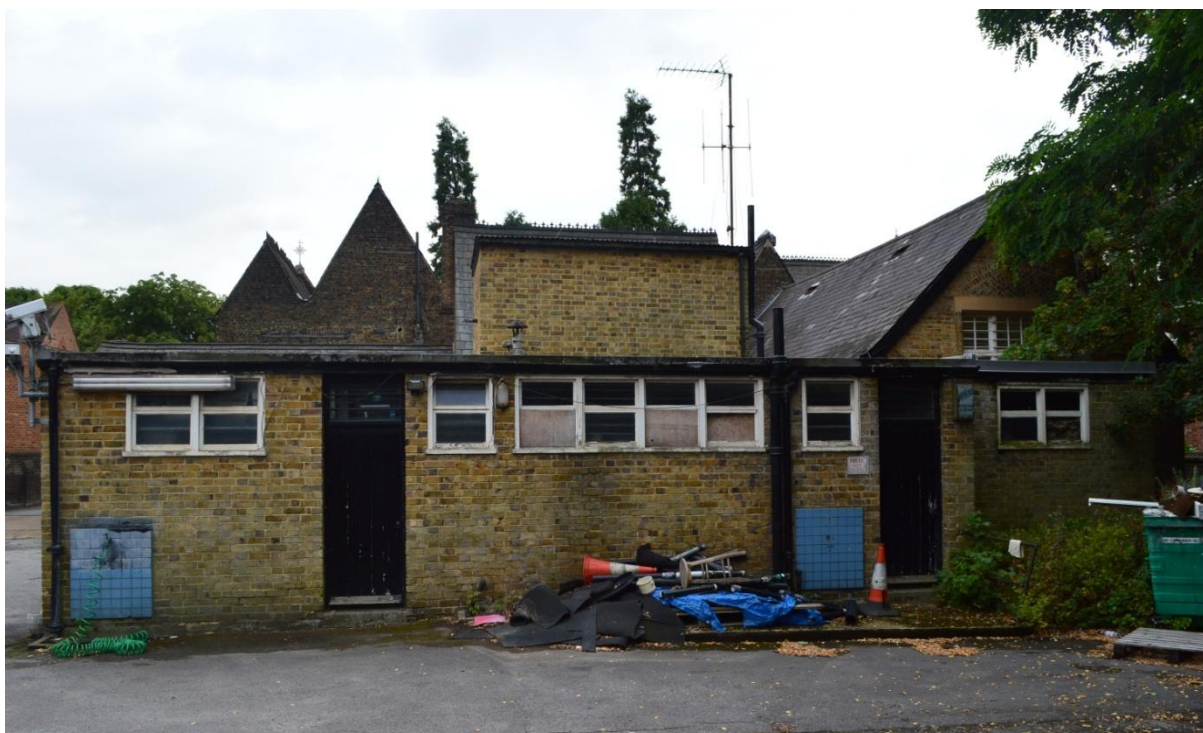
View from the north, showing the utilitarian 1950s extension which replaced the 1890s WC blocks. To the right is the upper part of the 1890s rear schoolroom extension.
