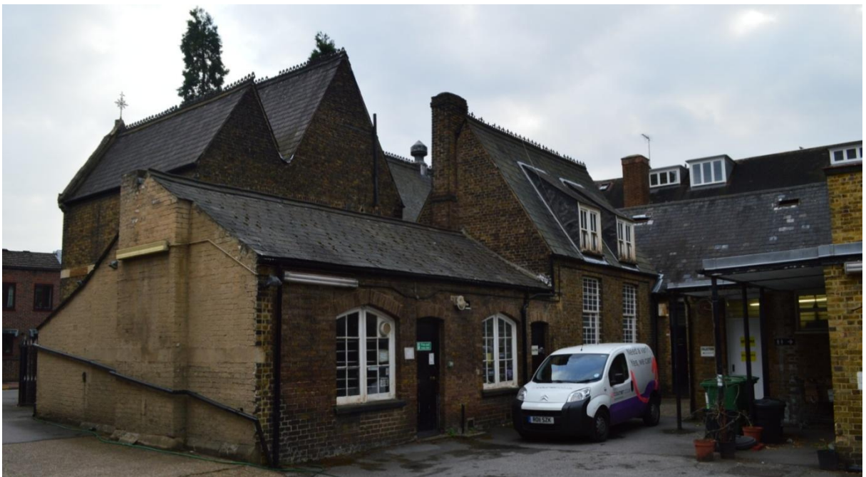
View of the rear of the original master's house (left) and class room (centre), with the roof of the 1890s rear wing on the right, above the 1950s extension.
