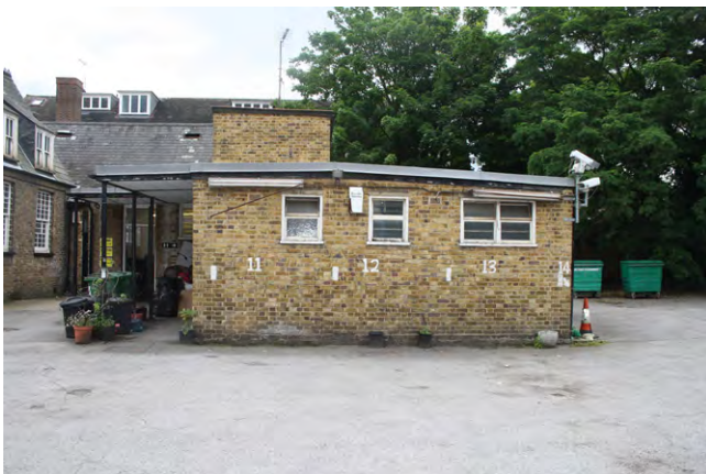
Plate 3. 1950s extension and surrounding playground/car park, looking west.
