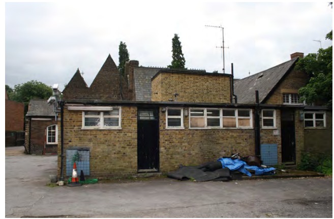
Plate 4. The school buildings with playground/car park in the foreground, looking south.
