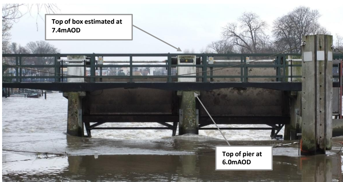
Figure 2-3 Picture illustrating position of white boxes above piers in baseline scenario
