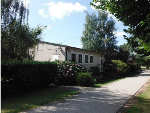
Figure 14 – Wooden building observed to be raised above ground on site
