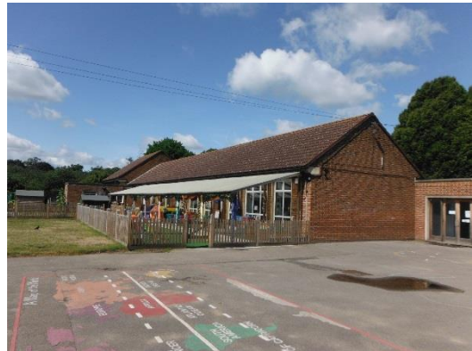
Figure 17 – View across playground to a school building in the south western corner of the site
