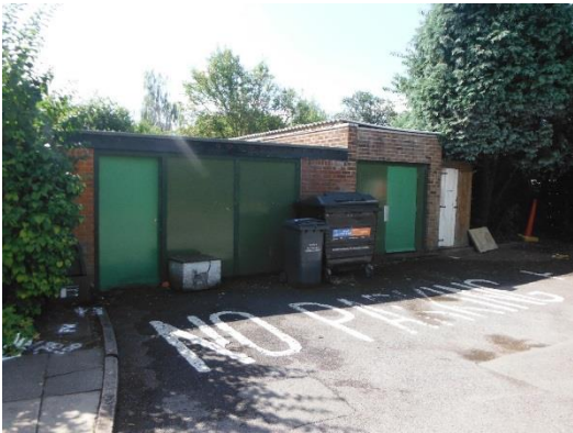
Figure 8 – Storage buildings near to school office
