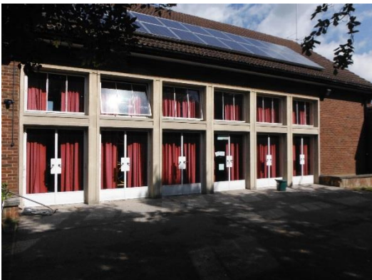
Figure 10 – School hall doors
