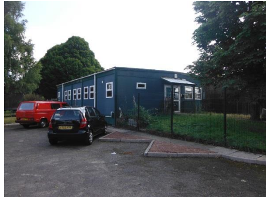
Figure 19 – Cabin building at northern boundary of Russell School
