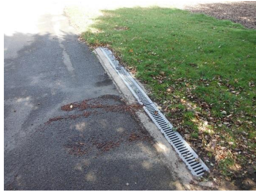
Figure 13 – Recently cleared drains serving the hard-standing Russell School playground
