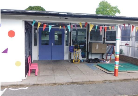
Figure 18 – Junior school building entrance
