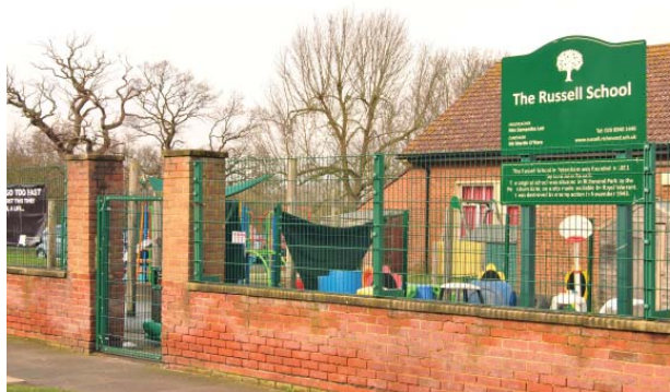
08 Access to the Infant Building (C)
