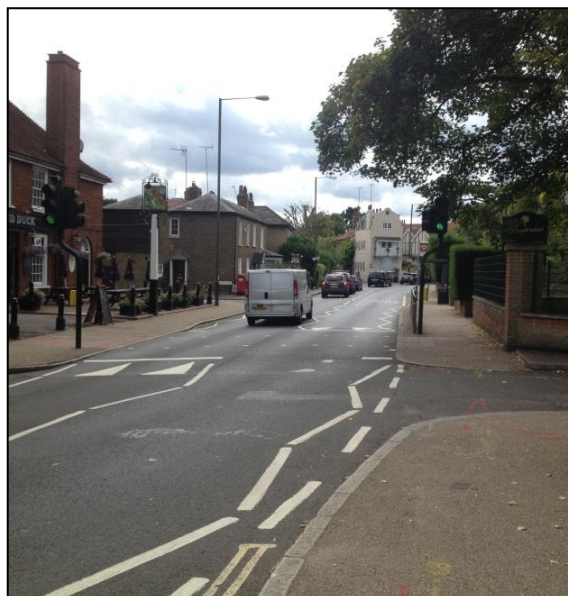
Figure 3.15 Southbound View of Petersham Road
