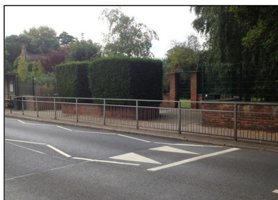
Figure 3.4 Pedestrian Entrance - Petersham Road
