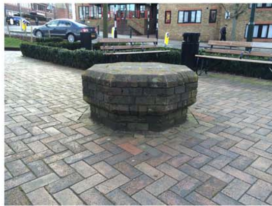
view of the brick plinth
