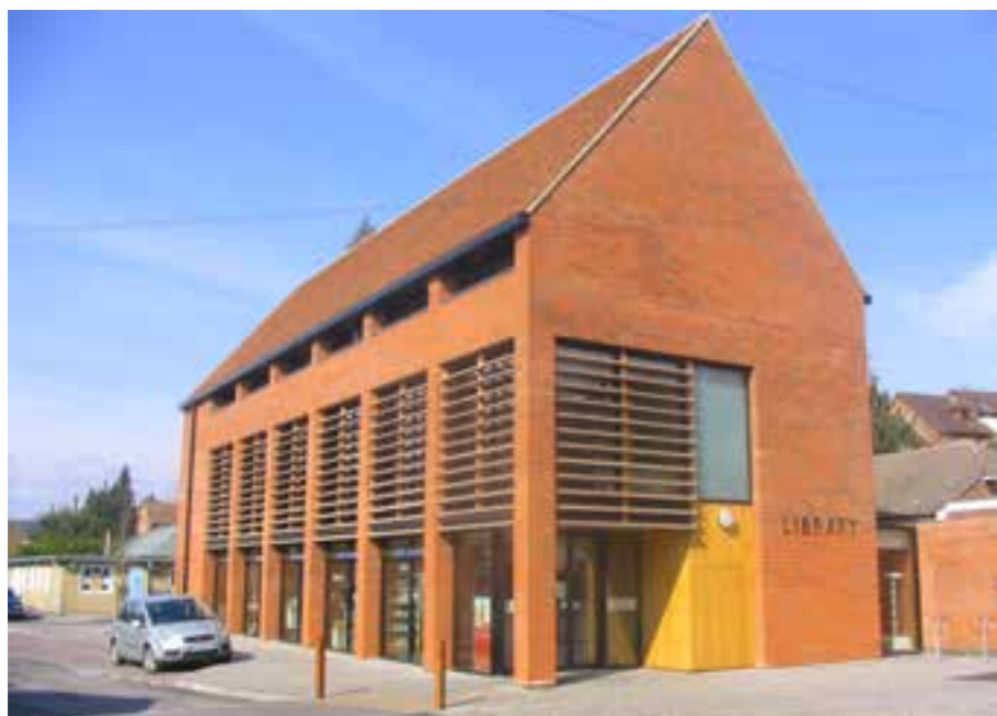
Architectural Inspiration - Alton Library, Alton, Hampshire, by Hampshire County Architects
