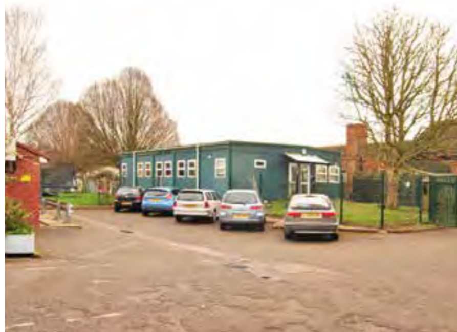
17 View of car parking area (A)
