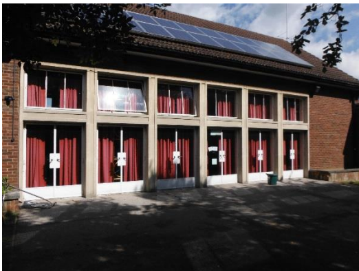
Figure 11 – School hall doors
