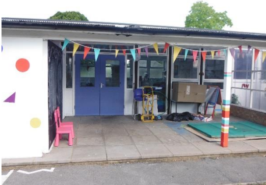
Figure 19 –Junior school building entrance
