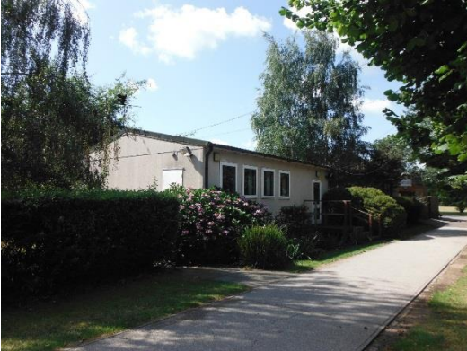
Figure 15 – Wooden building observed to be raised above ground on site
