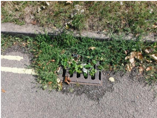
Figure 21 – Vegetated drain in Strathmore School car park
