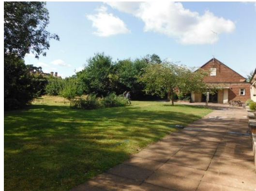
Figure 10 – View along the western face of the main school building
