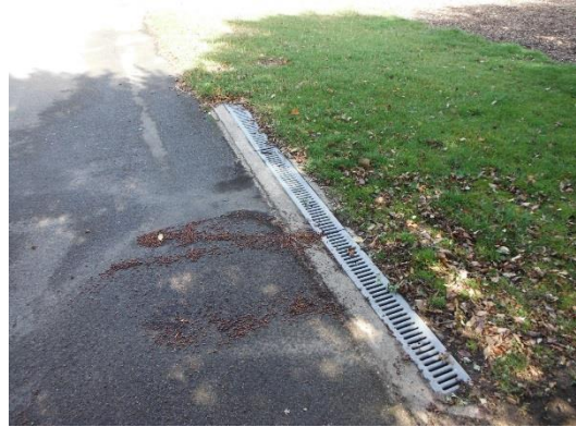
Figure 14 – Recently cleared drains serving the hard-standing Russell School playground
