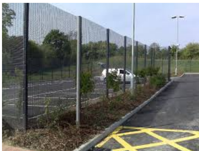
Figure 4: secure mesh fencing
