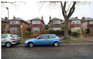
1. TYPICAL 1930S PRIVATE HOUSING ON CRANEFORD WAY.
