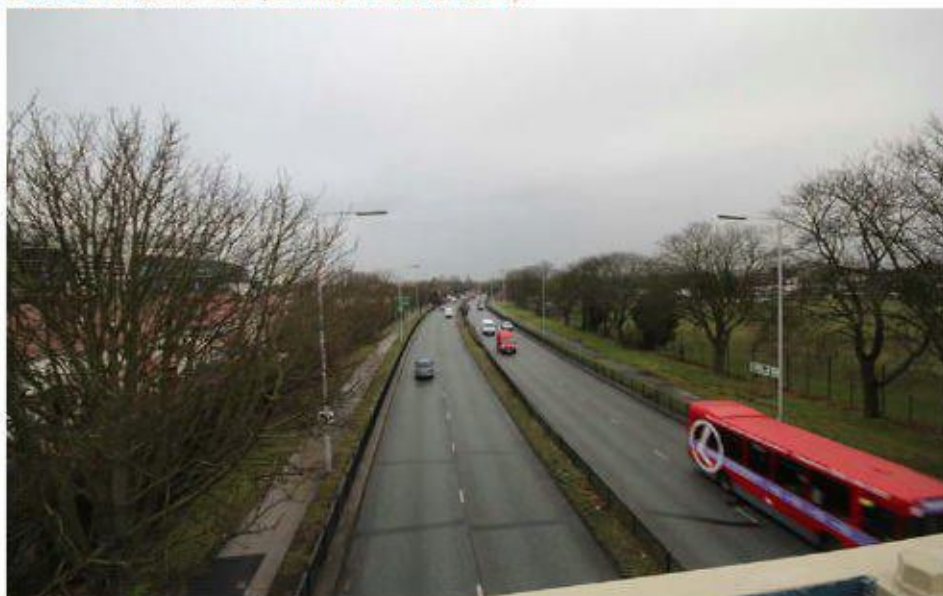
3. VIEW ALONG THE A316 FROM THE PEDESTRIAN OVERPASS SHOWING THE PROTECTED TREES TO THE NORTHERN BOUNDARY OF THE MAIN SITE.
