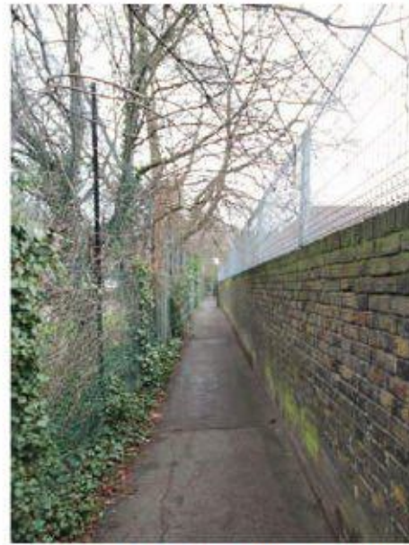
2. MARSH FARM LANE ALONG WESTERN BOUNDARY OF THE MAIN SITE.
