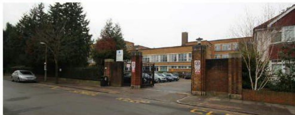
1B. EGERTON ROAD - PRIMARY PEDESTRIAN AND VISITOR ACCESS
