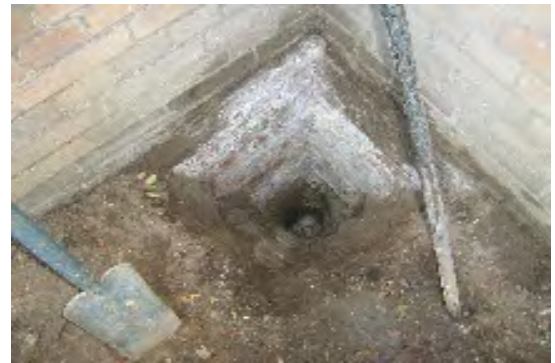
Photographic record of trial pit TP11
