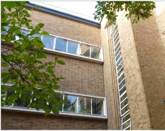
Photo 1 - gap between buildings
