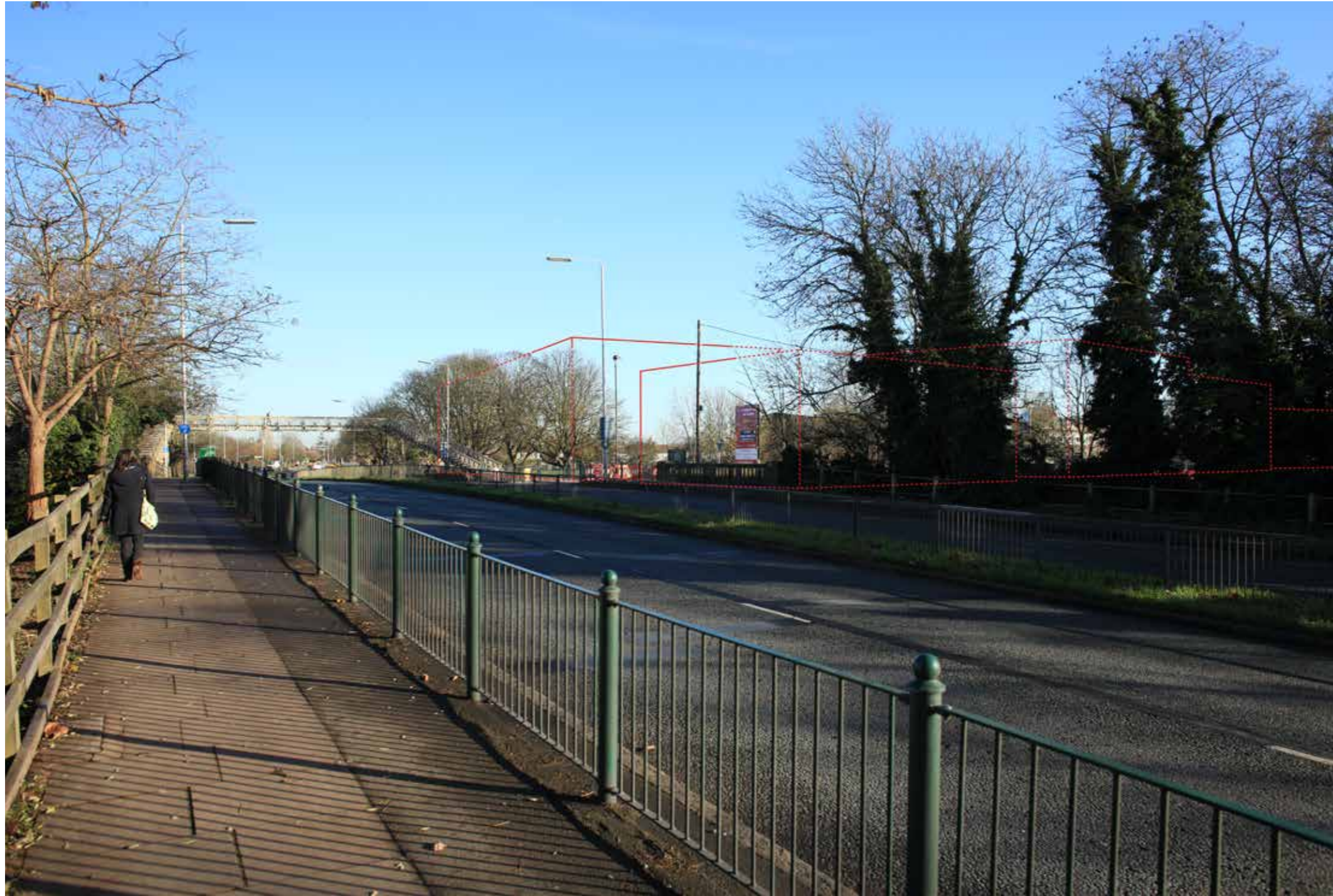
NB this image shows the the maximum parameters (built envelope) of the proposed buildings and the pedestrian footbridge has been removed. Details of the proposed works to the access are not shown.
