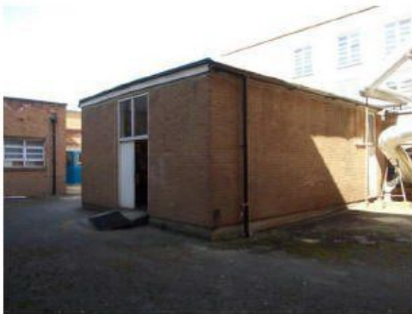
Photo 7: Richmond College Outbuilding
