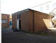
Photo 7: Richmond College Outbuilding
