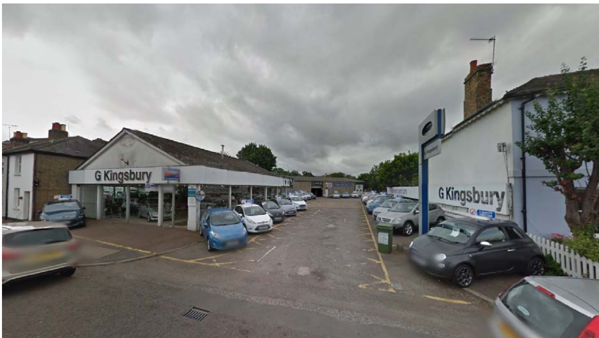
FIGURE 2: Existing Car Showroom, Station Road frontage
