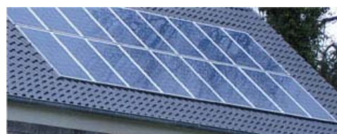
PV Panels semi-integrated to tiled roof
