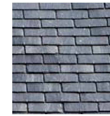
SLATE TILED ROOF
