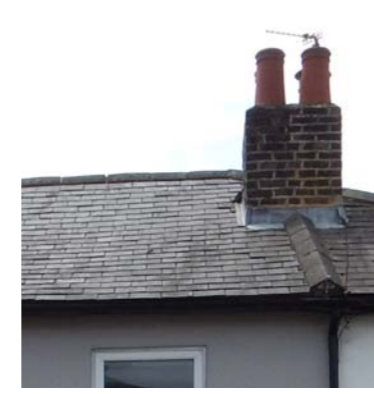
SHALLOW PITCH SLATE ROOF TILES
