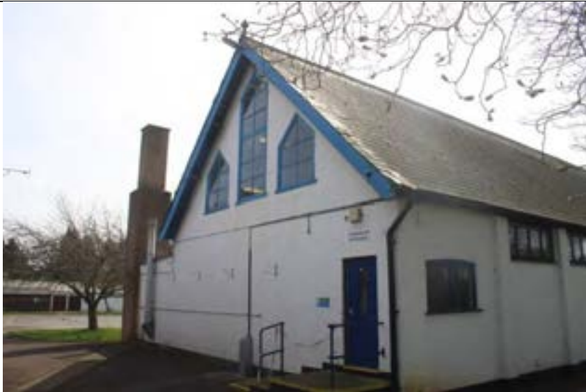
Plate 4. North-east aspect of Building 9 (gymnasium)
