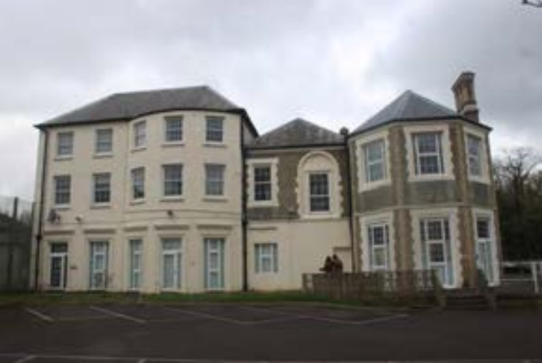
Plate 1. North facing aspect of the Building 1 (Main House)
