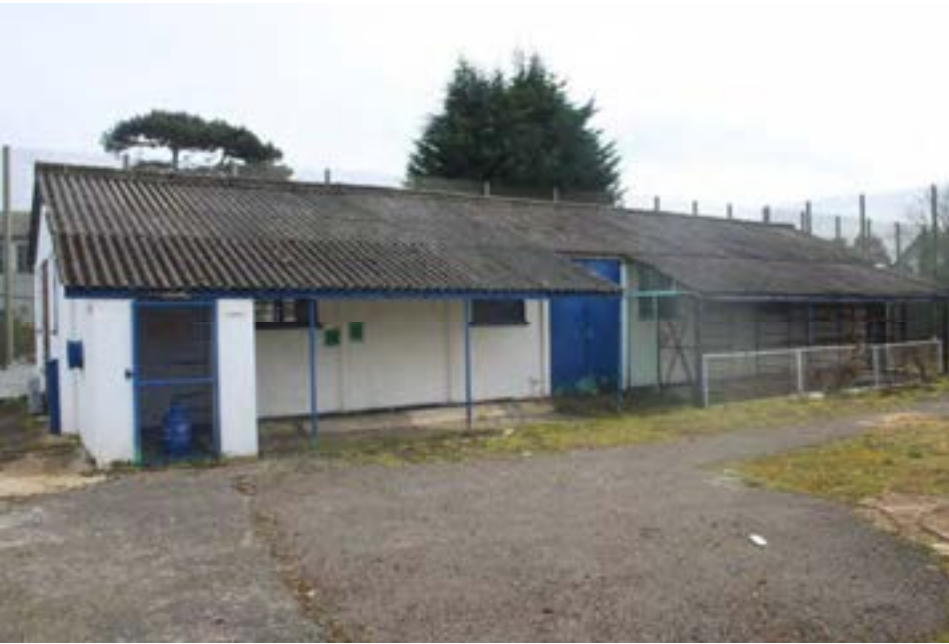
Plate 2. North facing aspect of Building 12 (workshop)
