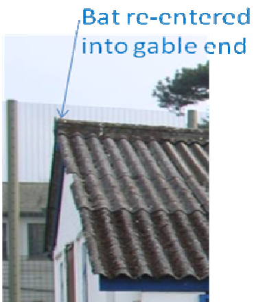
Plate 3. Bat access point at gable end of Building 12, re-entered 06/08/13.
