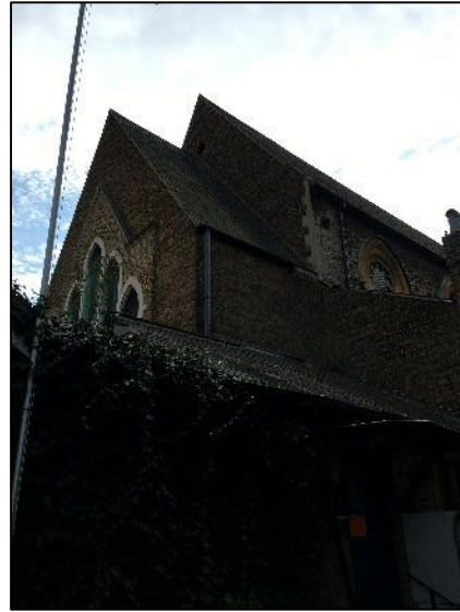
Photograph 2: Eastern elevation of church
