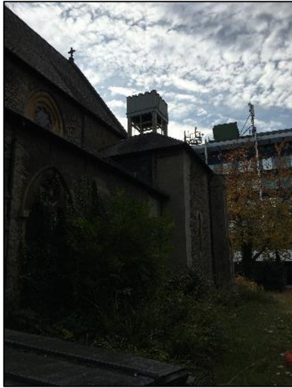
Photograph 1: Northern elevation of church
