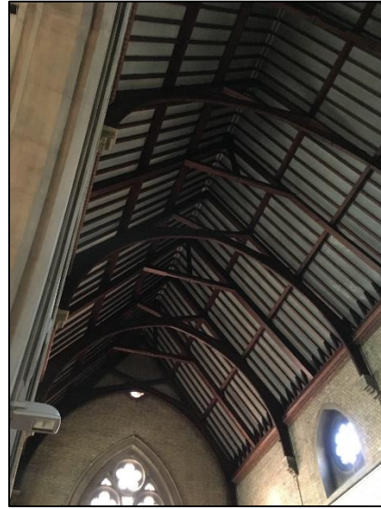
Photograph 10: Internal roof structure
