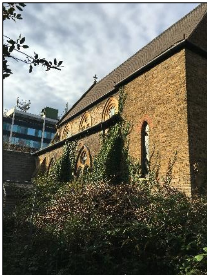
Photograph 3: Southern elevation of church
