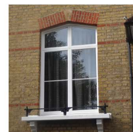
Photo 6: Red brick window head detail.
