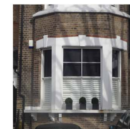
Photo 7: London stock brickwork with painted window surrounds.
