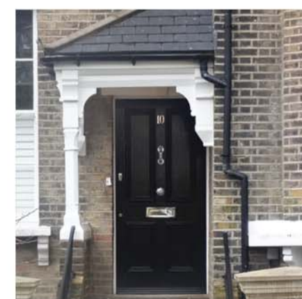
Photo 1: Intricate timber porch.
