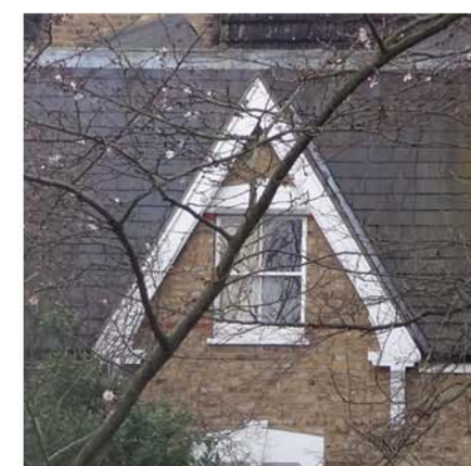
Photo 3: Slate roof with timber verge boards to gable end.
