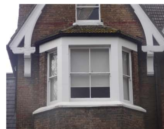
Photo 2: Decorative timber eaves detail.
