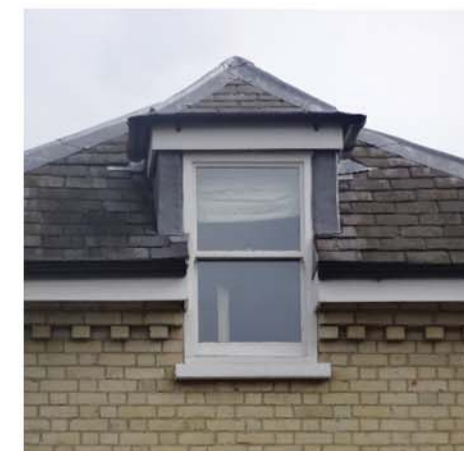
Photo 3: Lead lined dormers with timber fascia.
