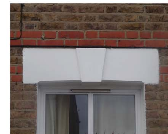
Photo 6: Rendered window lintel.
