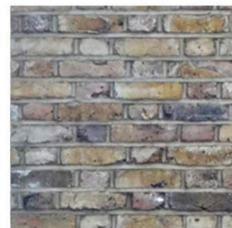
Photo 1: London stock brickwork.
