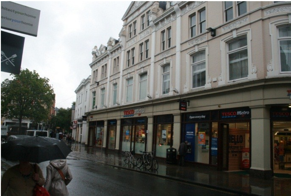
Figure 2: Site Photograph of 29 George Street, View from Petersham Road
