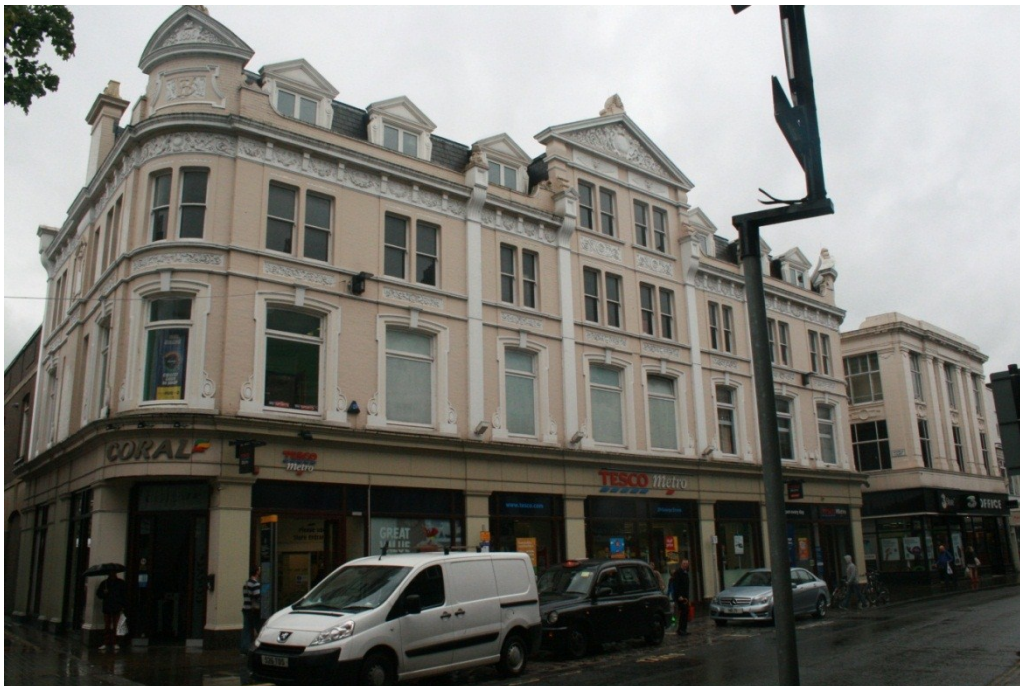
Figure 3: Site Photograph of 29 George Street, View from Petersham Road
