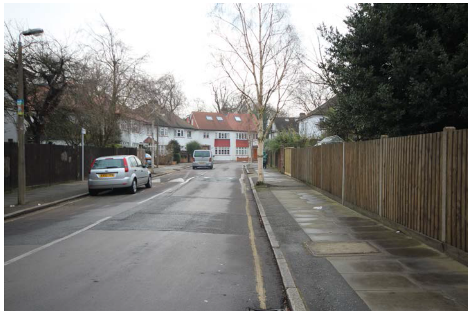
4. VIEW ALONG CRANEFORD WAY FROM COURT WAY.
