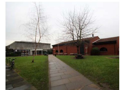
14. VIEW OF MUSIC CENTRE AND KLM BUILDING FROM MAIN BUILDING
