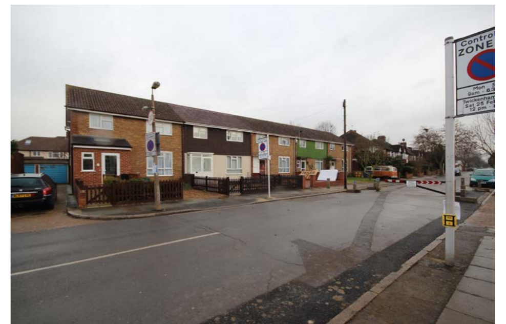
6. POSTWAR HOUSING ALONG EGERTON ROAD.
