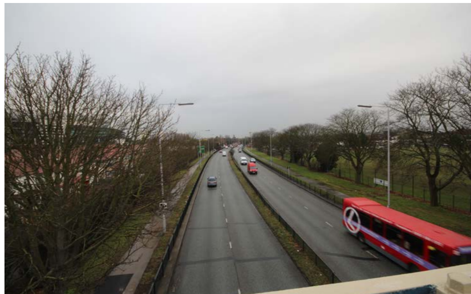
3. VIEW ALONG THE A316 FROM THE PEDESTRIAN OVERPASS SHOWING THE PROTECTED TREES TO THE NORTHERN BOUNDARY OF THE MAIN SITE.
