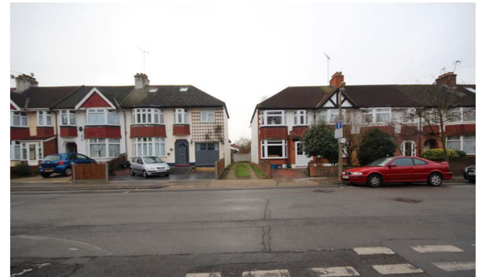
3. PRIVATE HOUSING ALONG EGERTON ROAD, SHOWING PASSAGE TO CAR PARKING BEHIND HOUSING.
