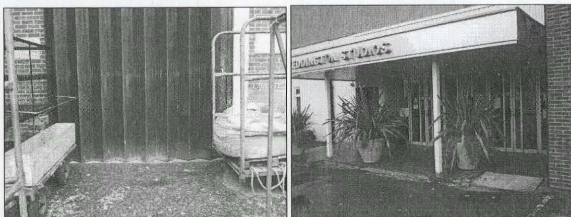
Figure 4-18 Selection of doorways and access points to buildings on the site
