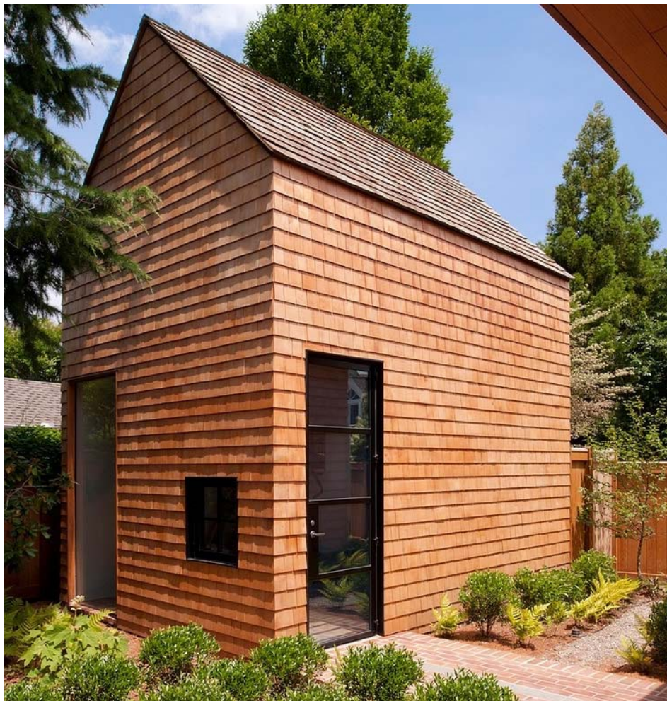
These pictures are not a computer generated images of the proposed house but are to illustrate how flexible cedar shingle are in their use.
