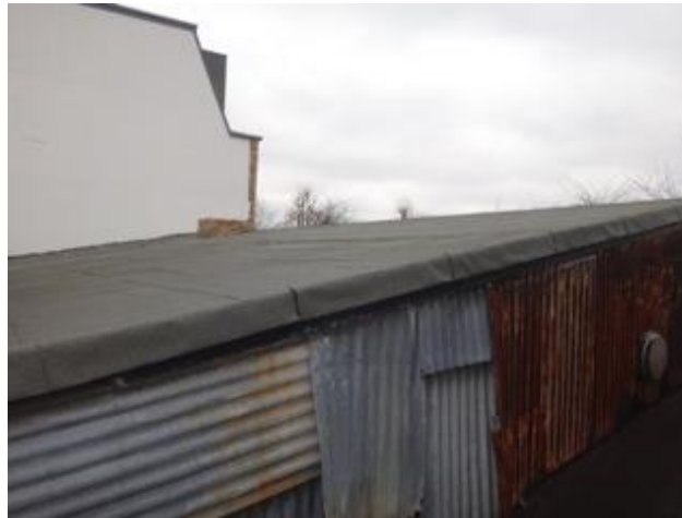
Photo 8- Roof and Southern Aspect of B2
