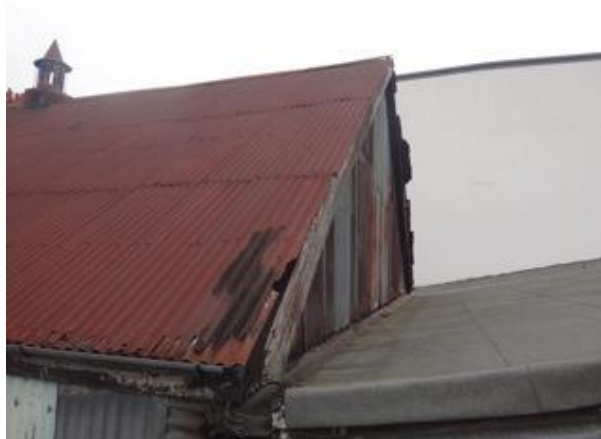
Photo 5- Eastern Aspect of B1
