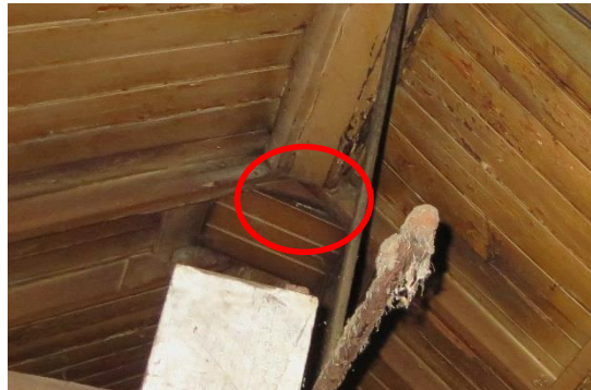
Photo 7- Small Access Hatch Leading to Open Chimney Vent
