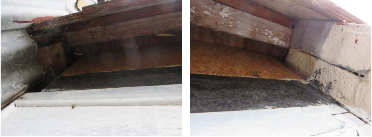
Photo 9 and 10- Potential Access Points above Door on Western Aspect
