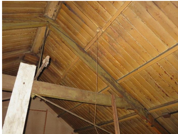
Photo 6- B1 Section 1 Loft Interior
