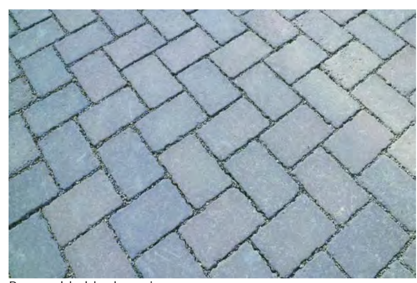
Permeable block paving
