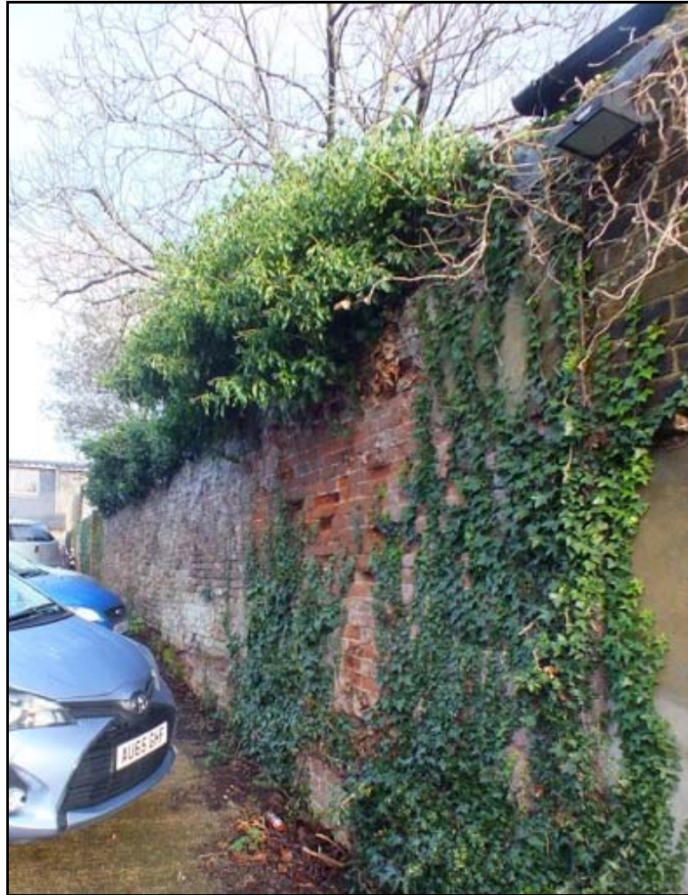
Plate 20: Eastern boundary wall in southern part of site, looking northeast.
