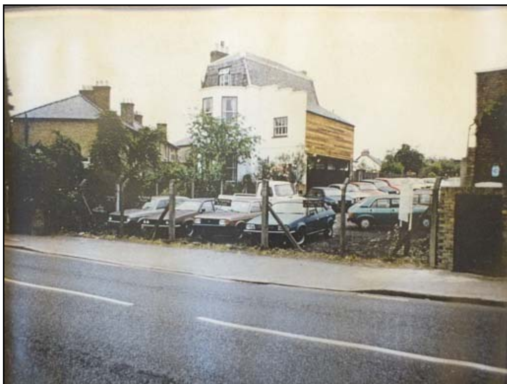
Plate 5: Site of Jessamine House post-1957 demolition (archive of G. Kingsbury & Sons Ltd.).
