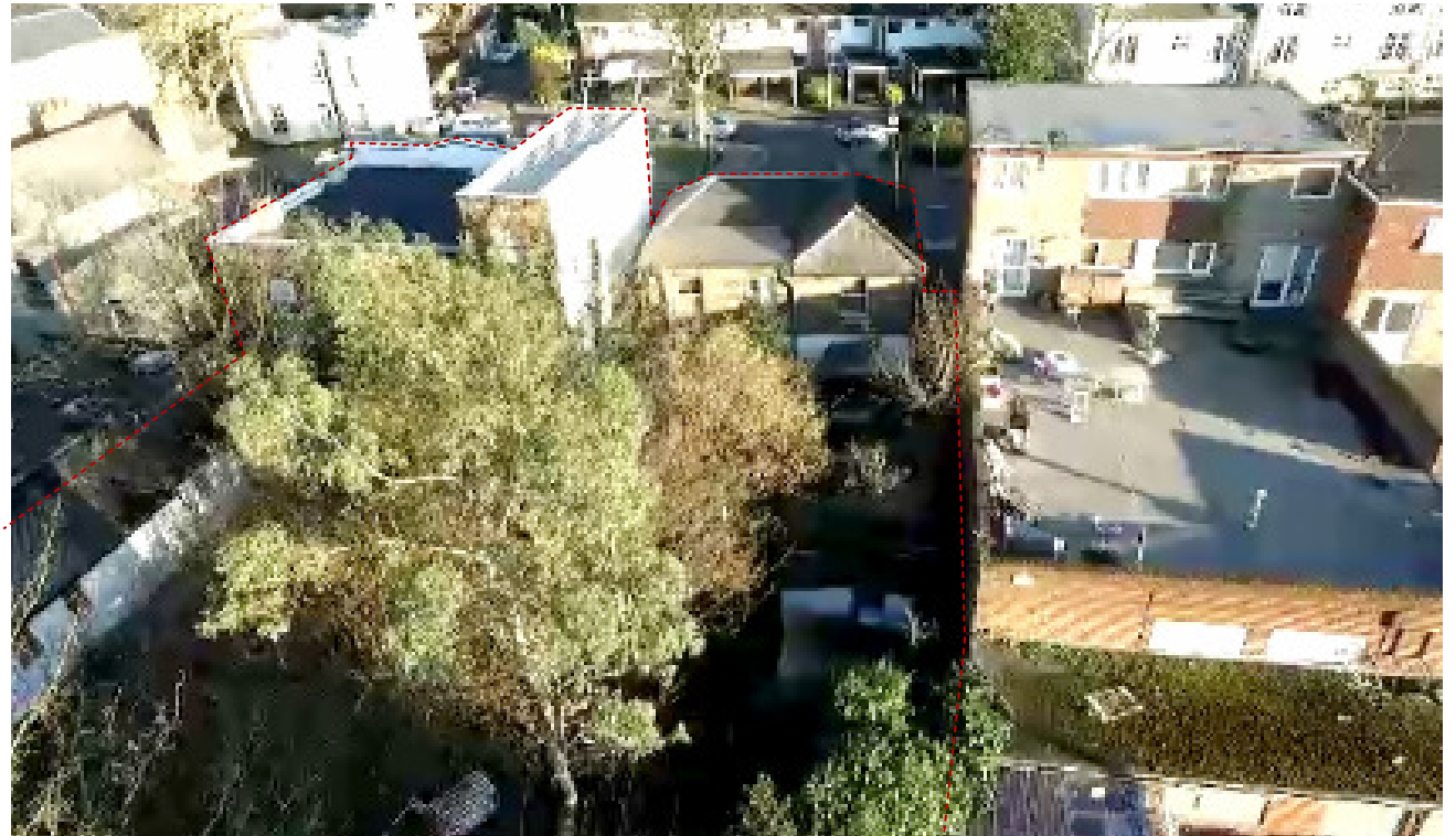
FIGURE 11 - AERIAL VIEW OF OVERGROWN AREA TO THE REAR OF THE EXISTING BUILDINGS
