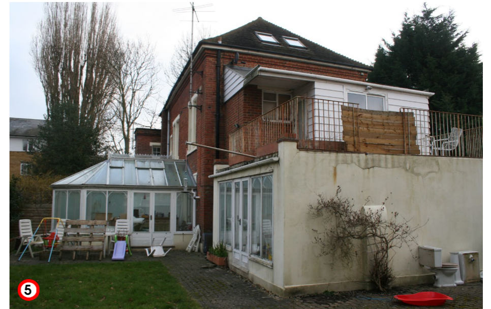
5 Poor quality additions
