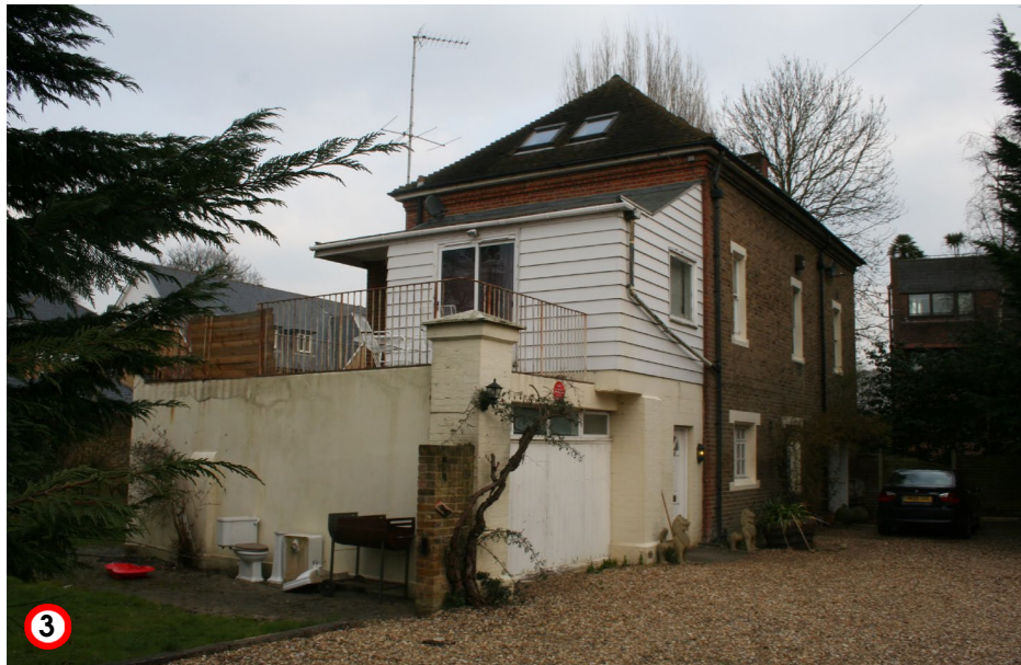
3 New extension to south west elevation
