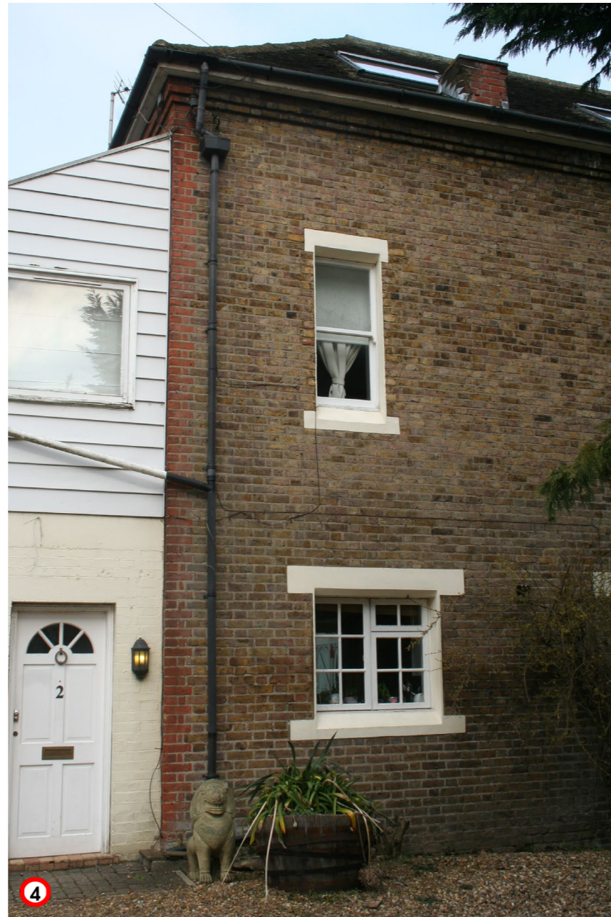
4 New windows to original part
