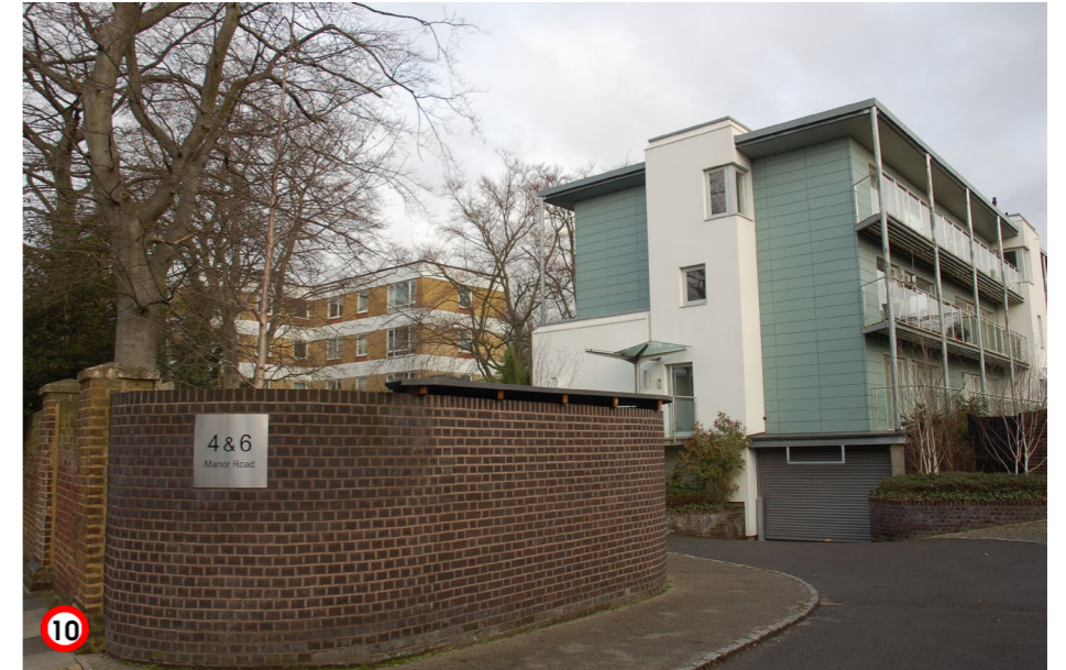
View of 4 Manor Road from street
