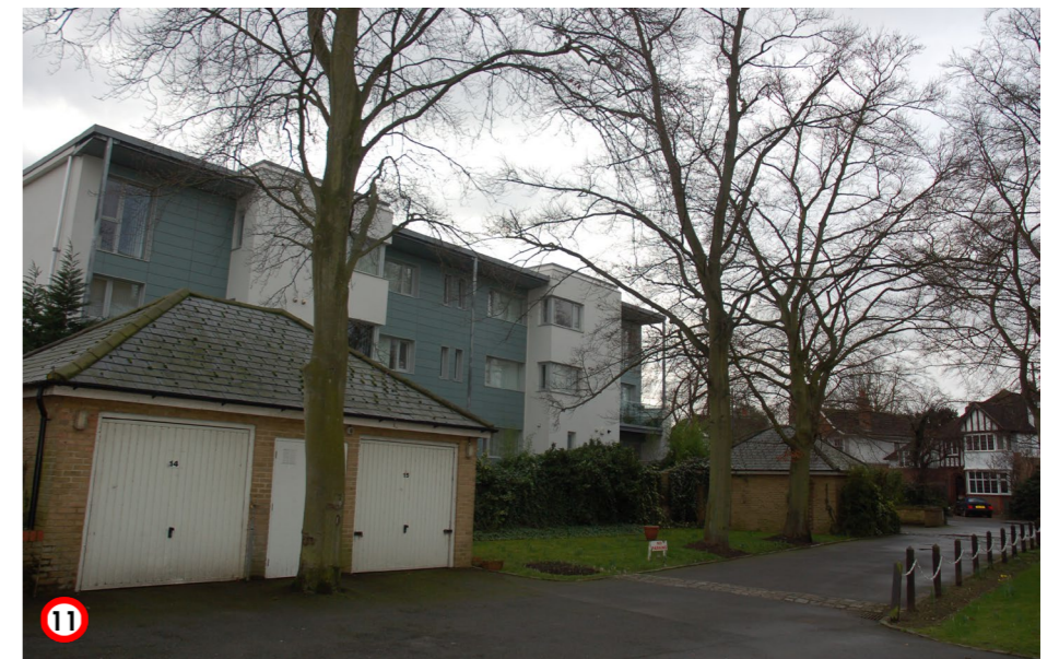
View of rear of 4 Manor Road
