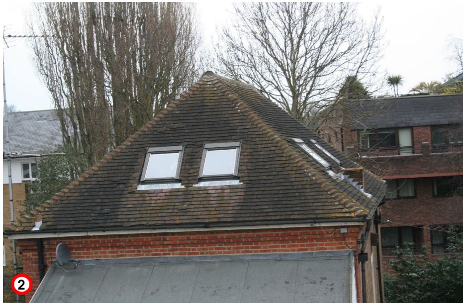
2 New roof fitted to original part
