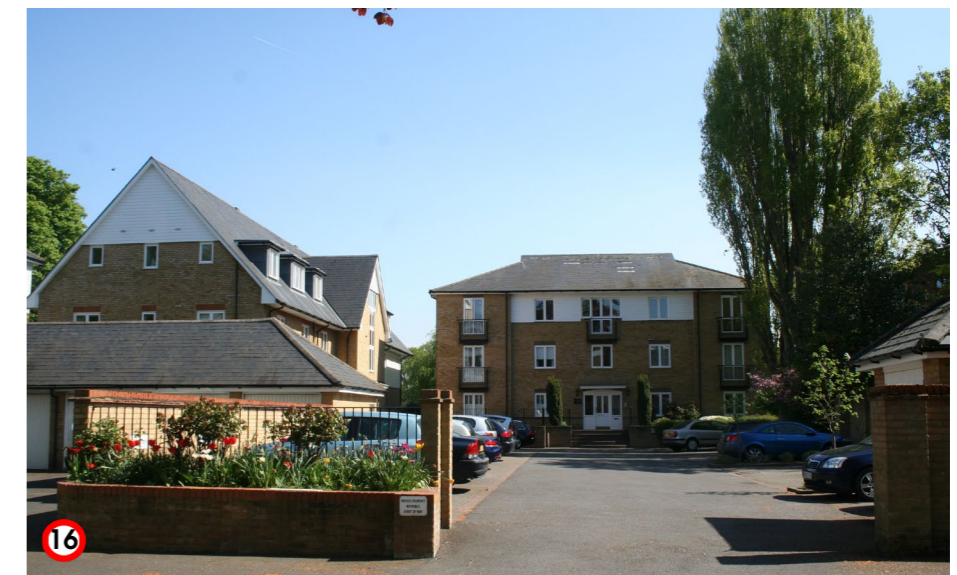
16 Duncombe House and Bowater House
