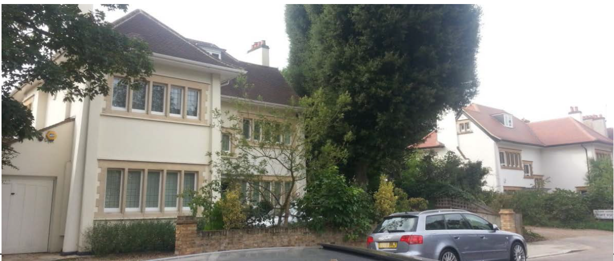
HEF JOB NO. 014 REF: 4 & 6 MANOR ROAD Figure 2: Roughcast render houses on Twickenham Road
