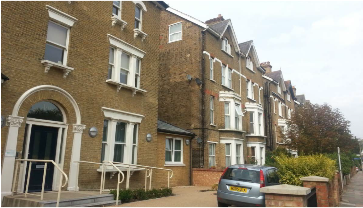
Figure 4: Semi-detached residences on Ferry Road
