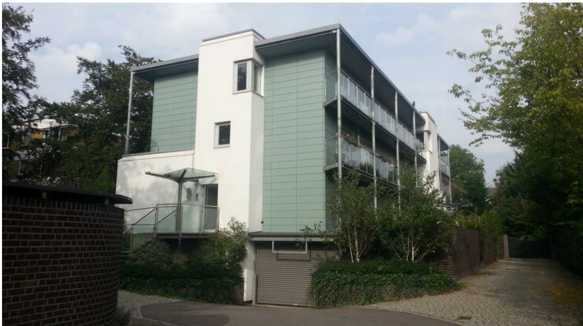
Figure 15: Photograph of existing building at no. 4 Manor Road
