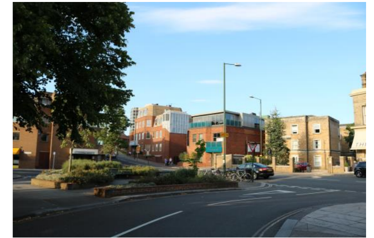
Plate 9: View from south-west from within Park Road Conservation Area
