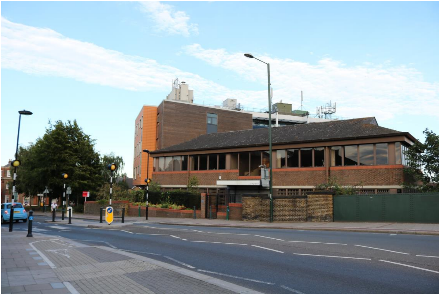
Plate 5: View of Informer House from north-west with backdrop of Holiday Inn
