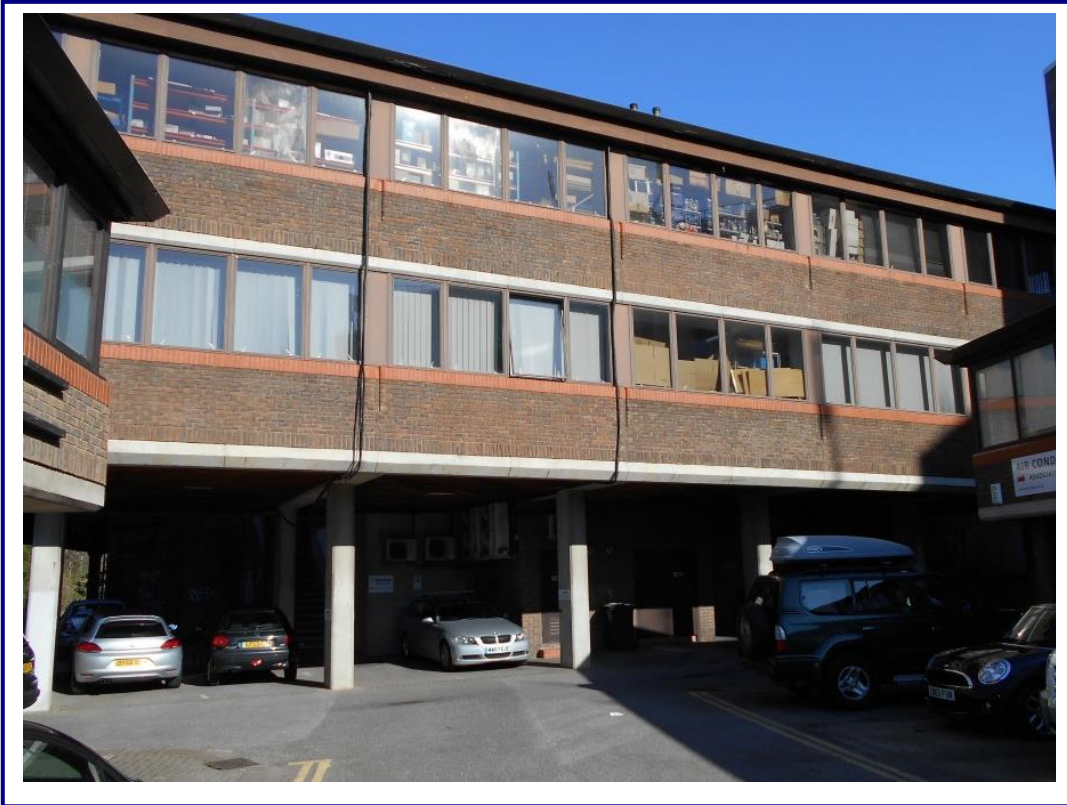
Photo 3: View from the rear of the site showing the undercroft car parking.
