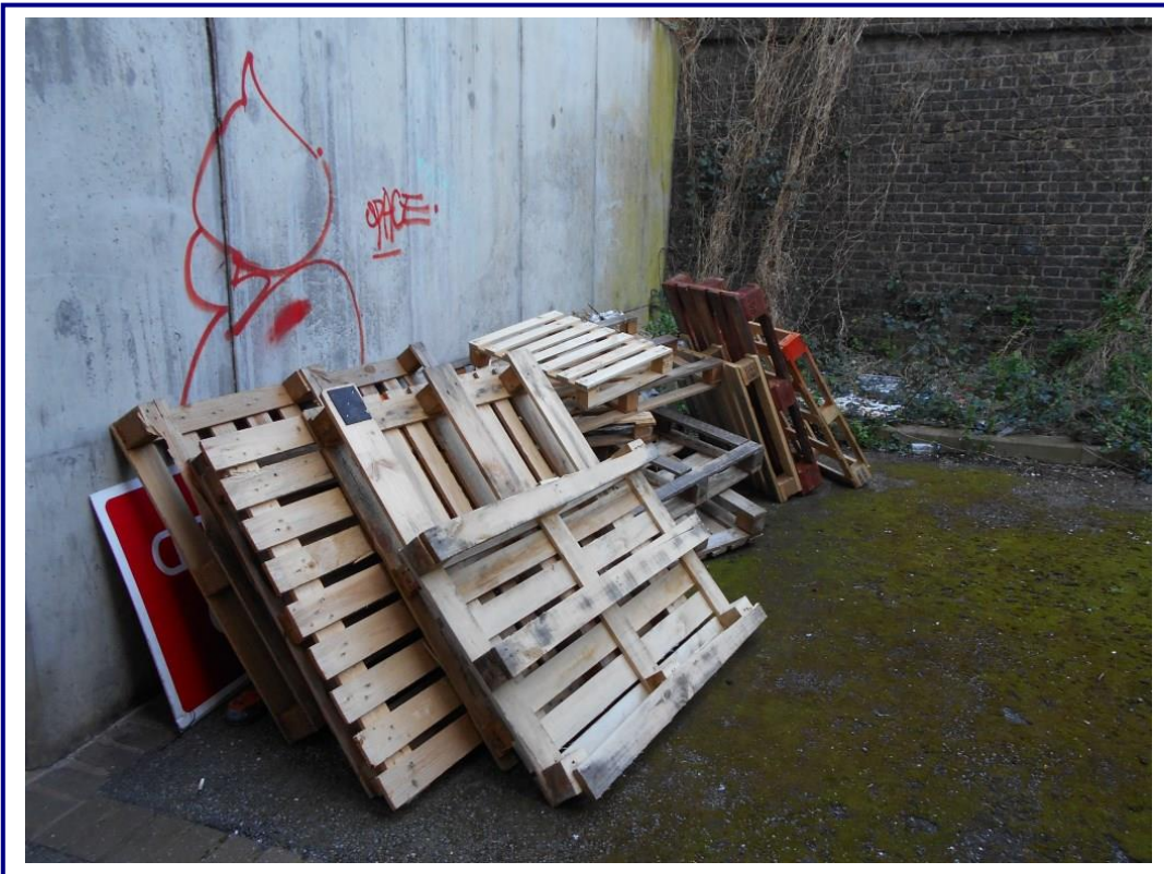
Photo 4: Pallets stored adjacent to the building at lower ground level.
