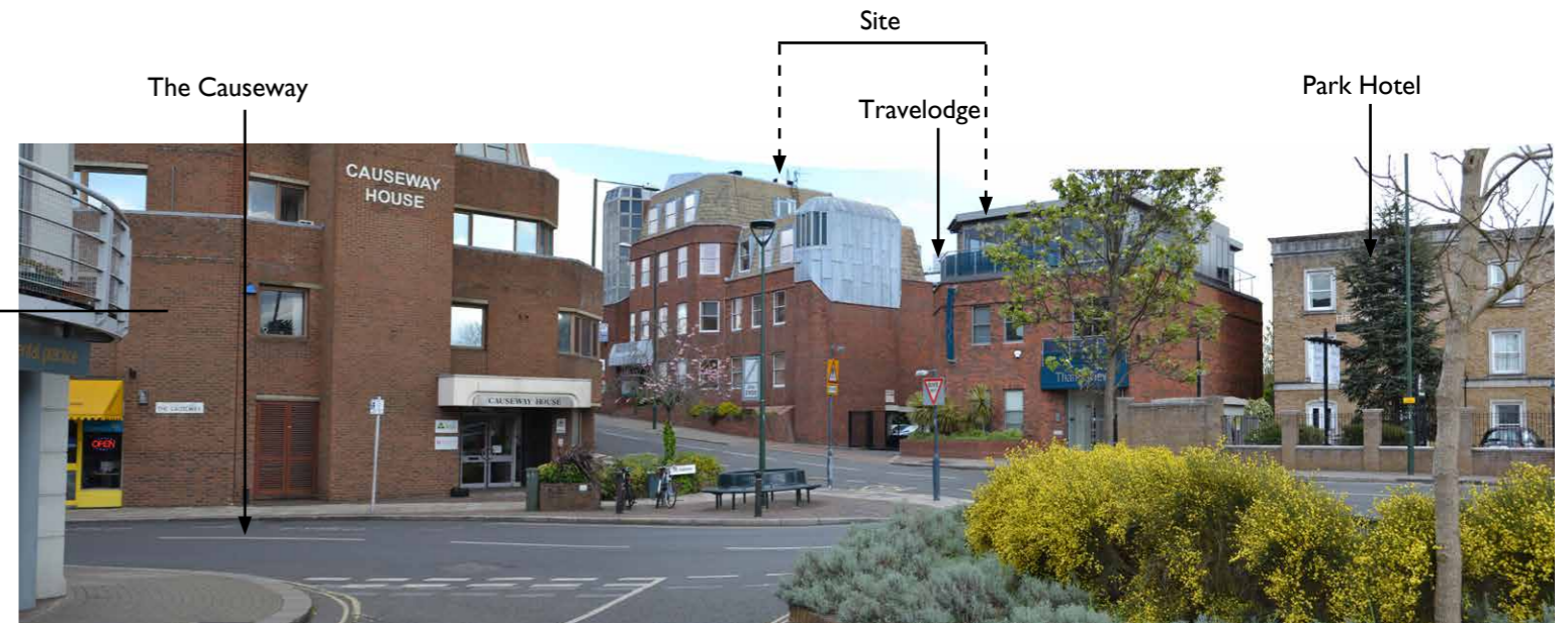
VIEW 10: Looking north-east
