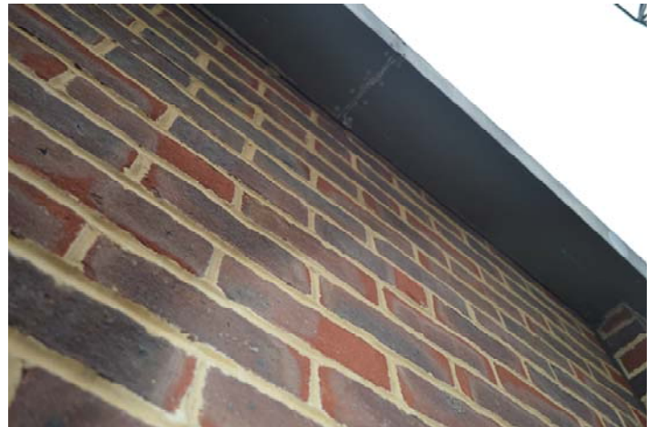
Photo 10 Metal cladding is generally tightly butted to brickwork with few bat access points
