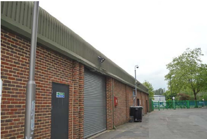
Photo 9 Maintenance Shed is single storey brick with metal clad roof
