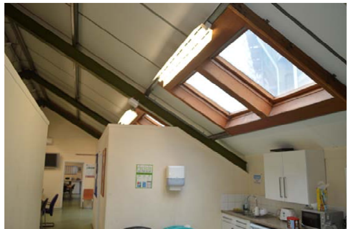
Photo 12 Internal view of maintenance shed
