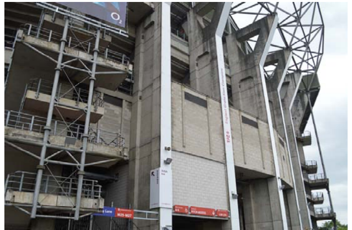
Photo 8 Some cosmetic fascias attached to concrete blockwork of East Stand
