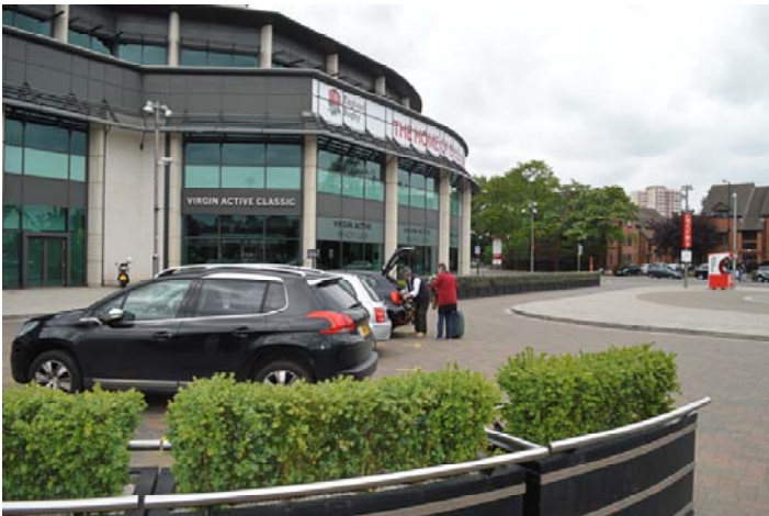
Photo 3 Hardstanding external concourse with movable planters
