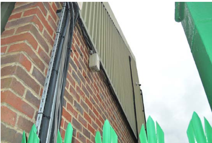
Photo 11 Maintenance shed Gable
