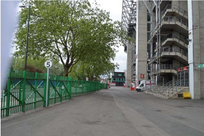
Photo 1 Concourse of East Stand with Street trees in Rugby Road slightly overhanging
