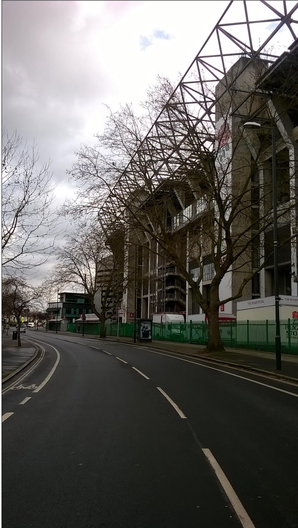
General site looking south along Rugby Road towards T2 and T3
