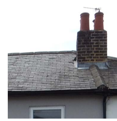
SHALLOW PITCH SLATE ROOF TILES
