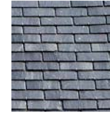
SLATE TILED ROOF
