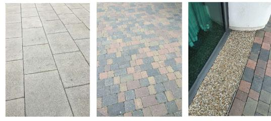
IMAGE 1 - EXISTING CONCRETE BLOCK PAVING AT SOUTH STAND
