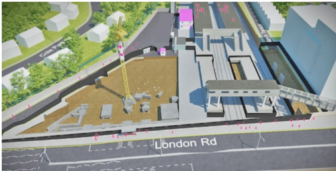
Figure 17 Block A pile caps piling – Tower crane and Mary's terrace pile caps
