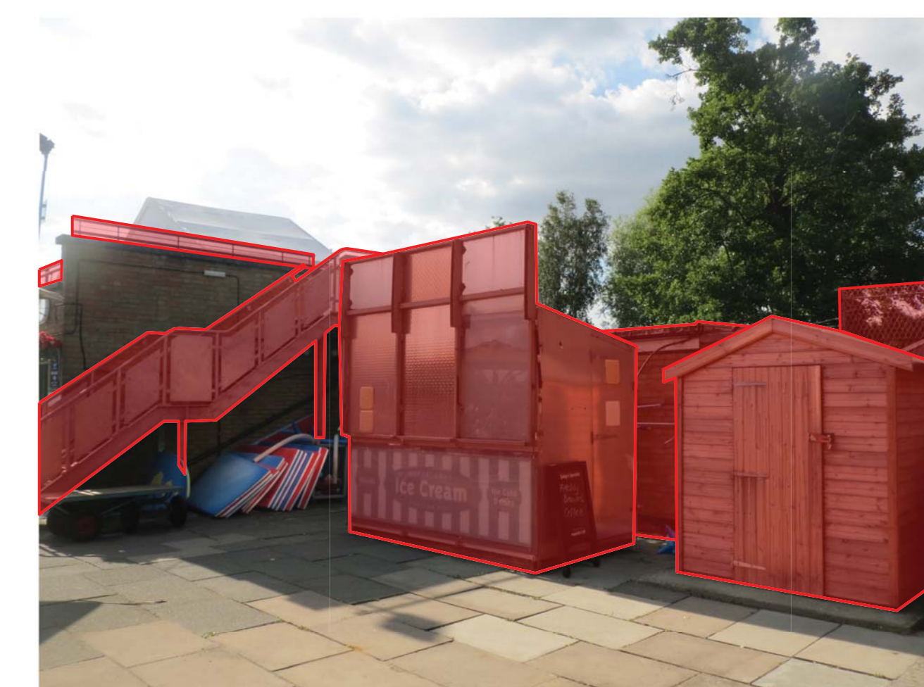
East end of existing building
