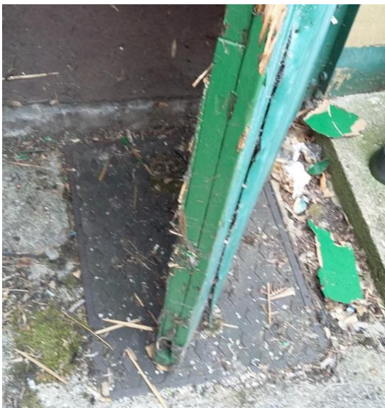
Photograph 2.4: Manhole cover located within the yard (foul sewer)
