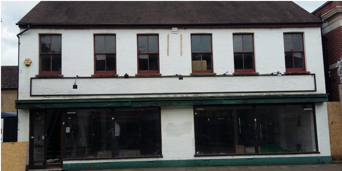
Photograph 2.3: Main building (149-151 Heath Road)
