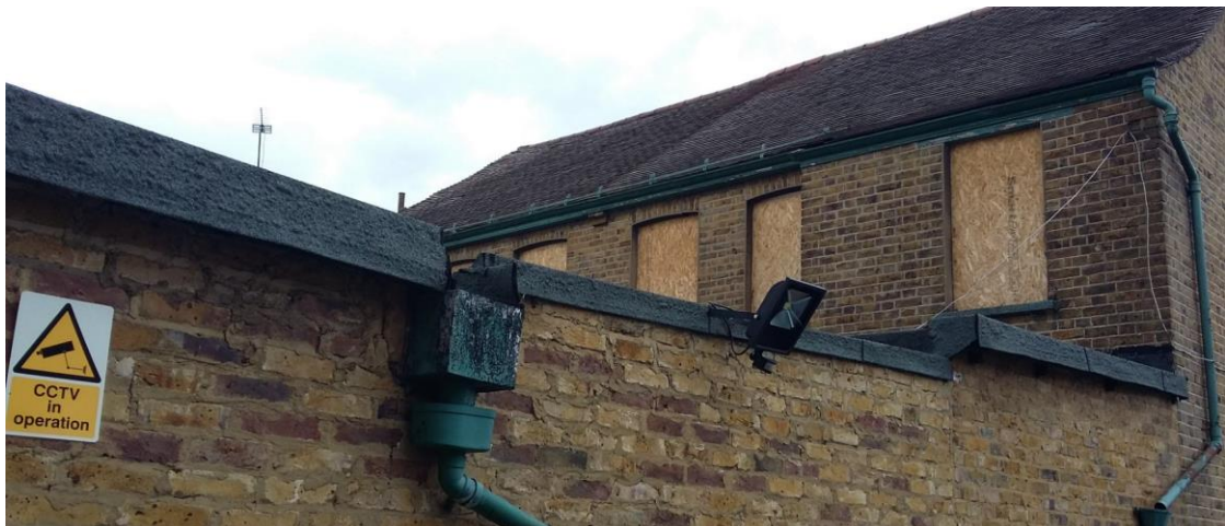
Photograph 2.6: Roof of single-storey store and two-storey main building
